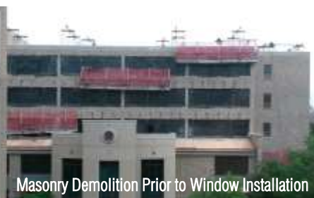
New Openings Cut / Masonry Work Progressing
